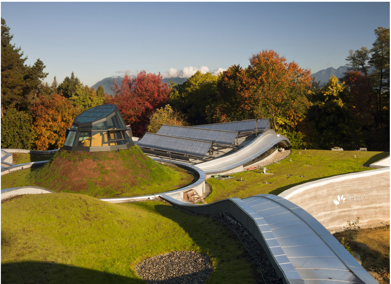
VanDusen Botanical Garden Visitor Centre Green Roof | Vancouver, British Columbia Photo: Nic Lehoux
