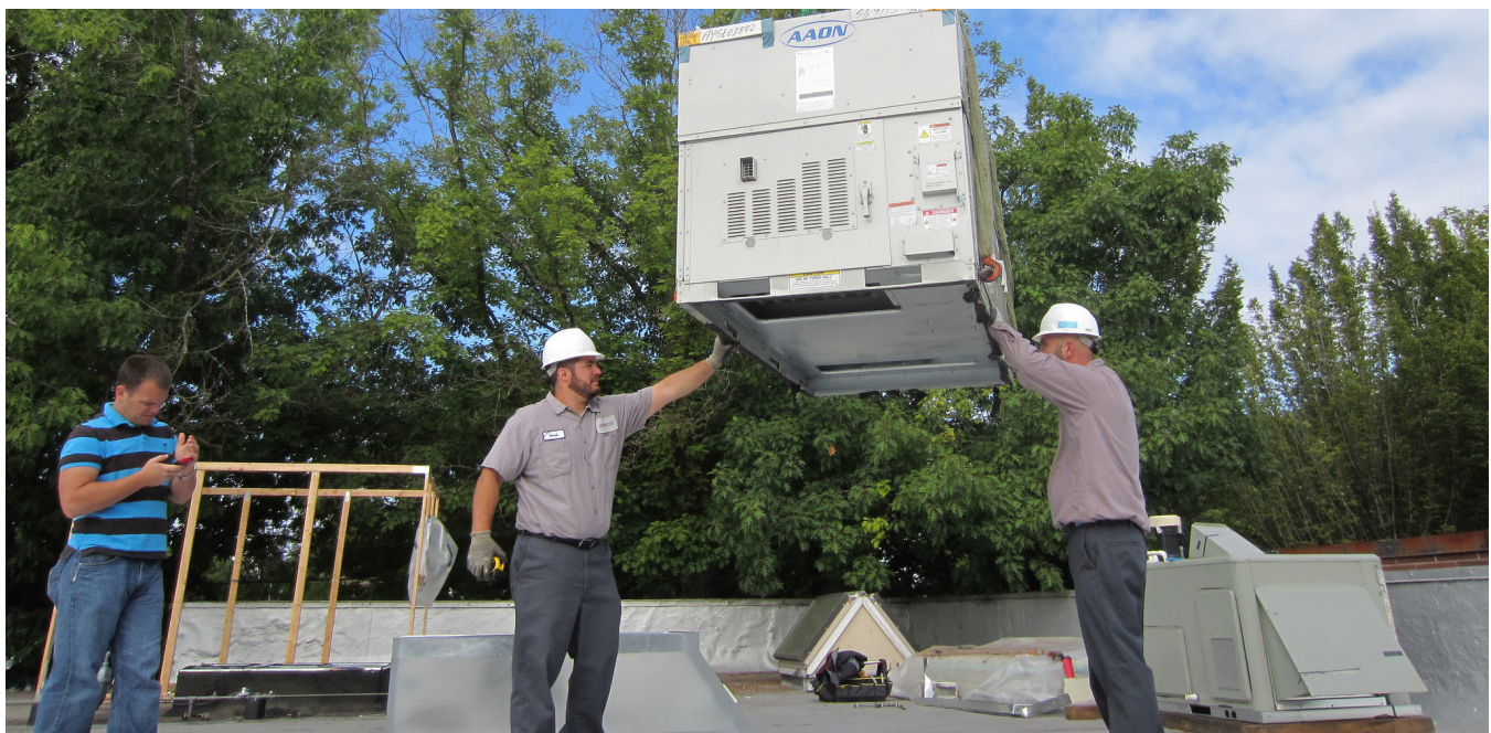
Installing a new HVAC unit | Vancouver, WA
