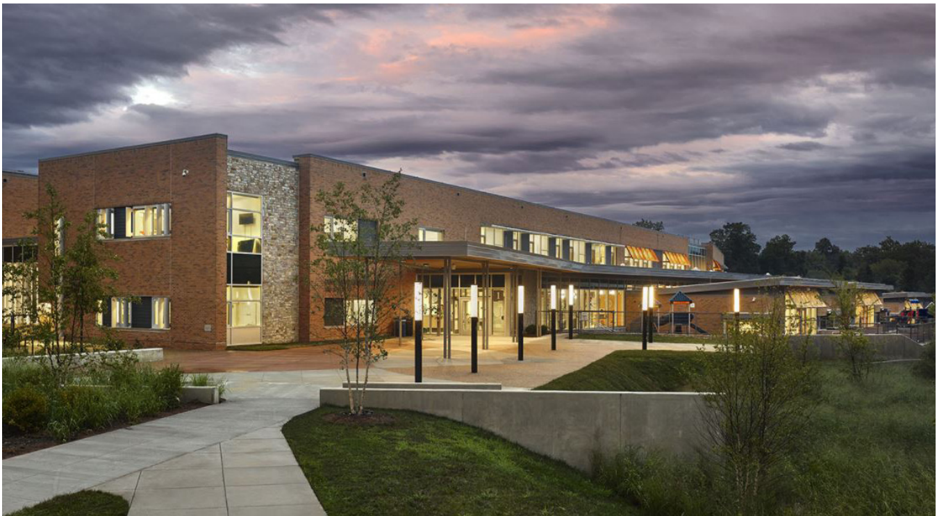
Discovery Elementary School | Arlington, VA Photo: VMDO Architects
