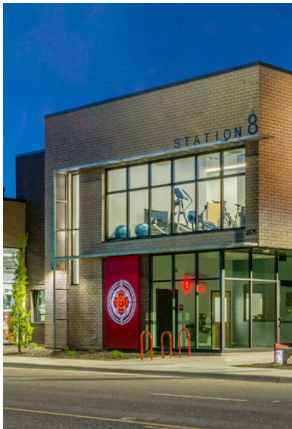
Fire Station 8 | Boise, ID Image: Cole Architects
