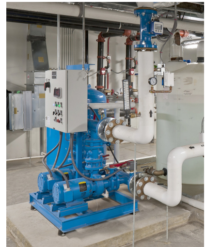
Turkey Foot Middle School Rainwater Catchment System | Edgewood, KY Photo: Piaskowy and Cooper Architects
